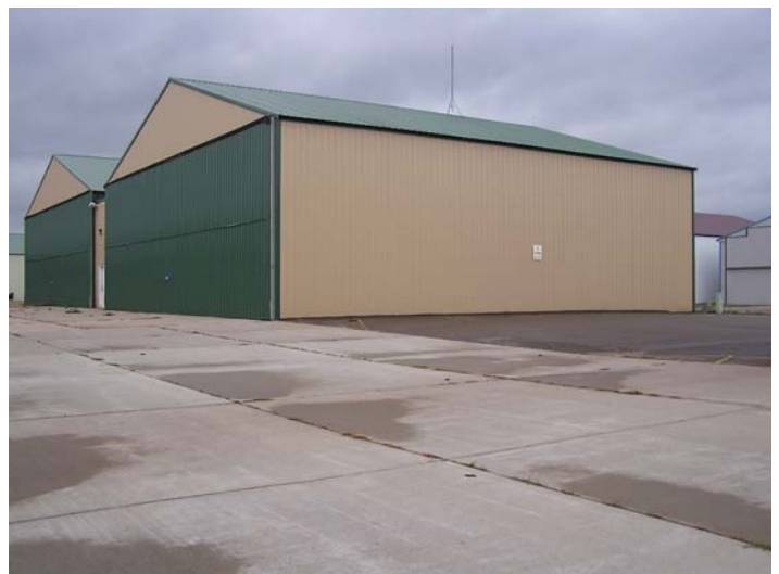
Hangar Plus Vehicle Parking
